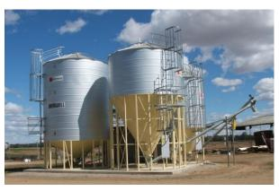
Grain milling complex with Skiold 2500 disc mill, 15T finished product silo, 75T cereal silo and 50T protein meal silo with out-load augers.
